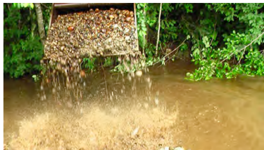
Photo 10 – Cleaning close to the berms
