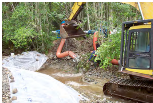
Photo 15 - Plastic-lined dam and second pumping station – Cleaning the intake screens
