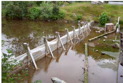
Photo 5 – Outlet plastic-lined dam
