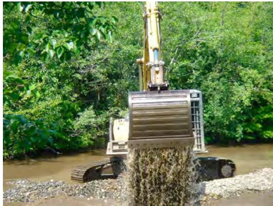
Photo 9 – Scoop and recast cleaning method
